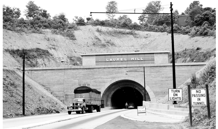
Laurel Hill Tunnel, Pennsylvania Turnpike, July 1942. Raised median divided traffic. (Library of Congress)
