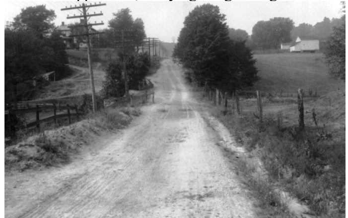
Cumberland road 1½ miles west of Brownsville, Pa , 1911 Packed-gravel macadam surface remnants visible a century after laid. (John Kennedy Lacock, Library of Congress)
