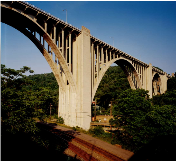
On the Lincoln Highway (US. 30), in East Pittsburgh, the George Westinghouse Bridge – world's longest concrete arch span in 1932 – arcs 240 feet above the Monongahela Valley, over Pennsylvania Railroad's tracks to Philadelphia. (Historic Amer. Engineering Record, Library of Congress)
